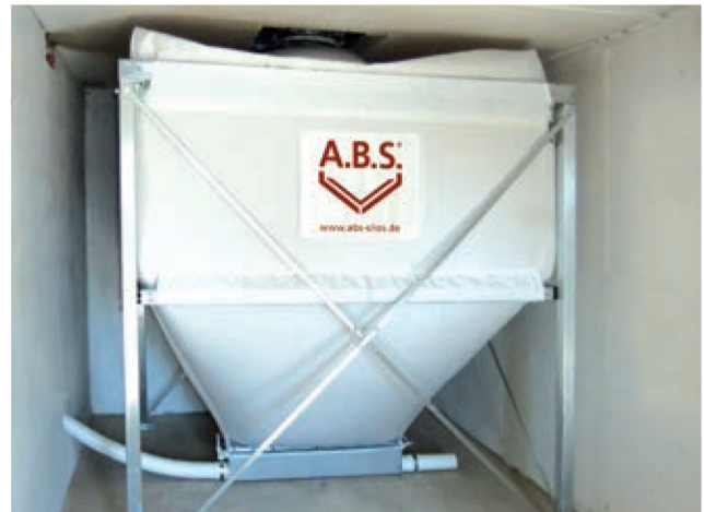
Flexilo trough with textile cone and spiral for direct feed
