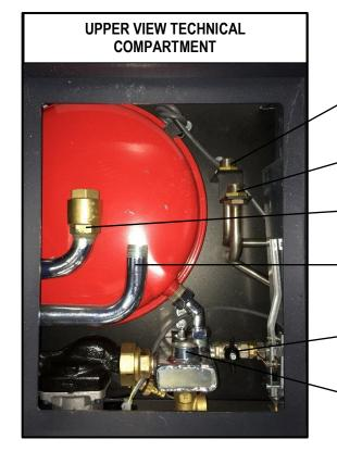
Domestic hot water outlet pipe connection (on prepared models only).
